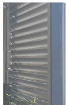
Existing Veranda structure to be reused
